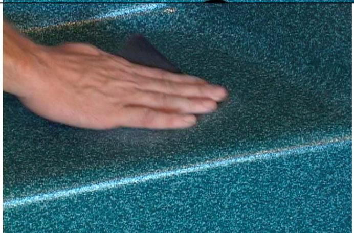
Now you are ready to apply the protective, clear topcoat. We recommend using only the K2000 product since it withstands the effects of spa water and chemicals. The required components include a hardener, thinner/reducer, and the topcoat.
