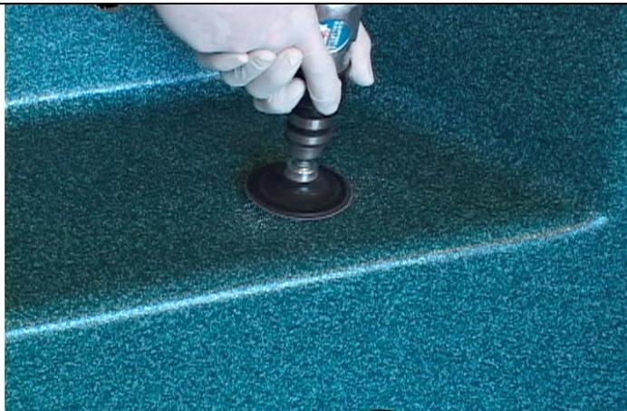
6) Sand the surface to the desired smoothness using a progression from 100 to 320 grit sandpaper.
